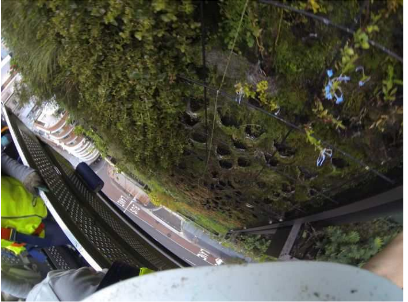
Image: Plants are planted within felt slits in the wall. (Ann Jones)
