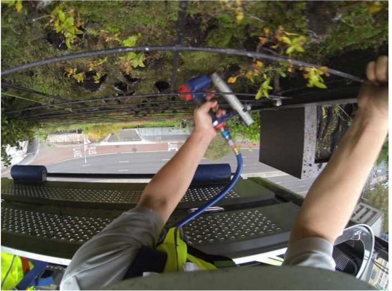
Image: Plants are stapled in place high above the Sydney Streets. (Ann Jones)
