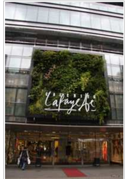
The vertical garden at the entrance of Galeries Lafayette in Berlin where the plants have to be chosen based on their tolerance of the cold weather
