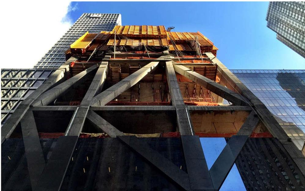
“The irregular structural pattern of crisscrossing beams,” according to CityRealty, creates a curtain wall made of “non-mirrored glass and painted aluminum elements, and along the tower’s mechanical and ventilation areas, a secondary system of mullions and louvers adds further depth.”
