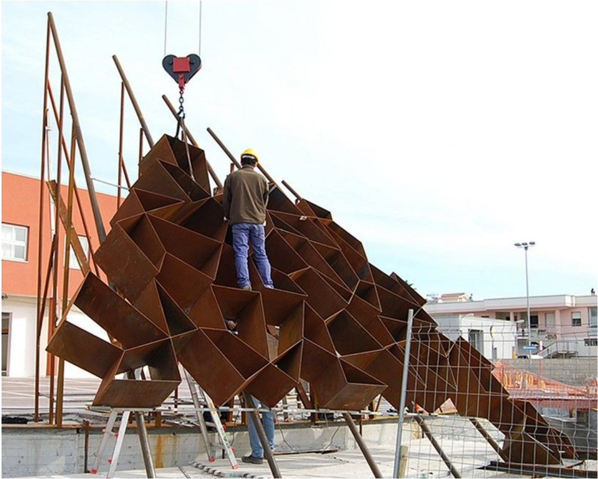
an individual part is lifted by crane
