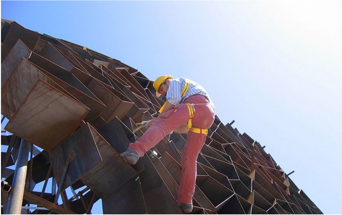
the construction is welded together
